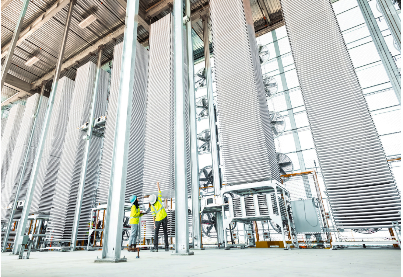
Two Heirloom technicians inspect a row of contactor towers in Heirloom's commercial Direct Air Capture facility
