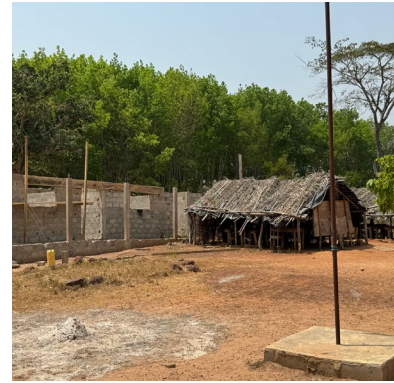
A school under construction with VSLA support in Petit-Paris.
