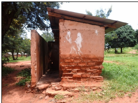
Typical school latrine
