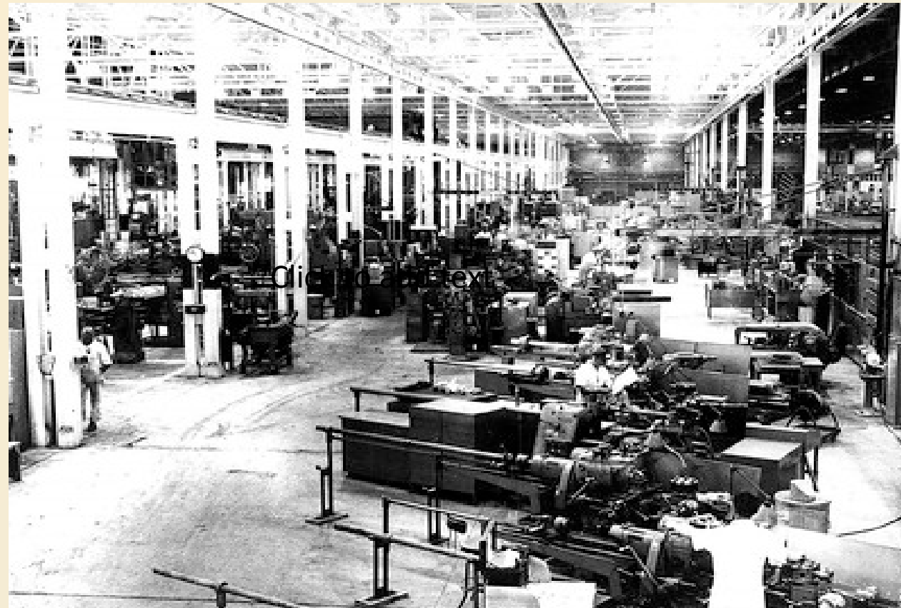
Oak Ridge Gaseous Diffusion Plant – Machine Shop
